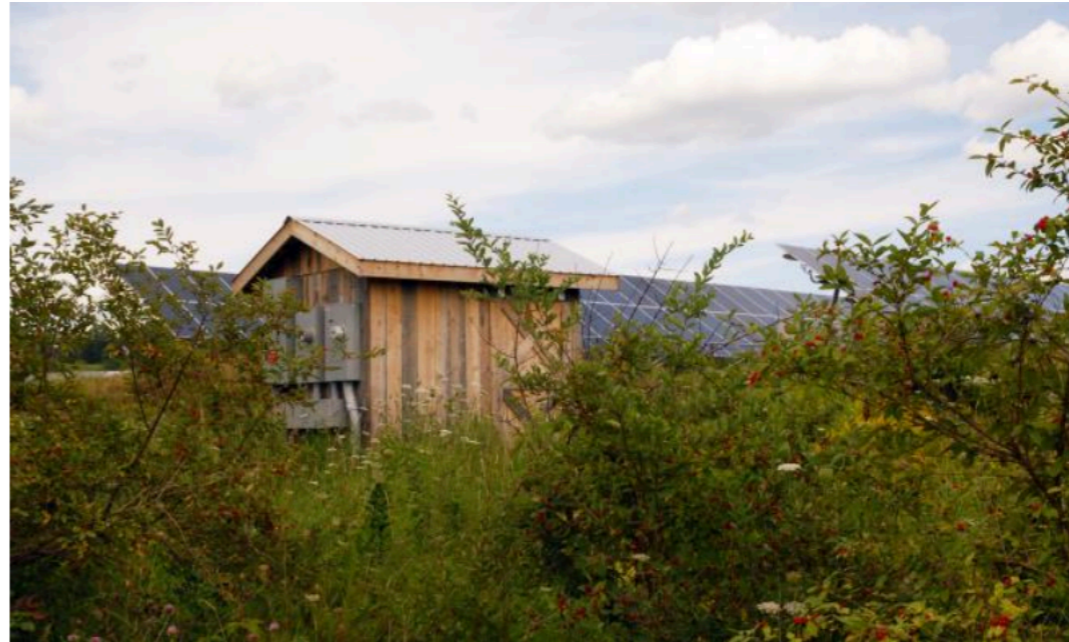
McKnight Farm 100kw solar array, screened from Kelton Road (Jean Vissering)
